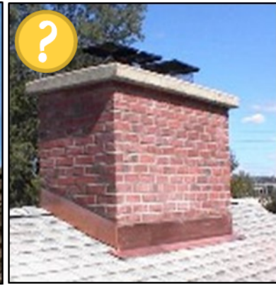
Brick Chimney with black metal flue caps
