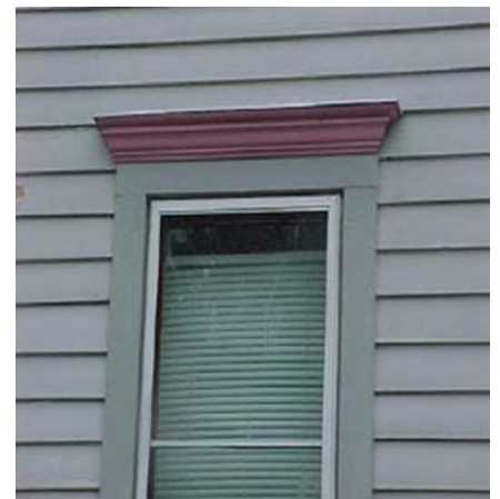
Window cap molding detail
